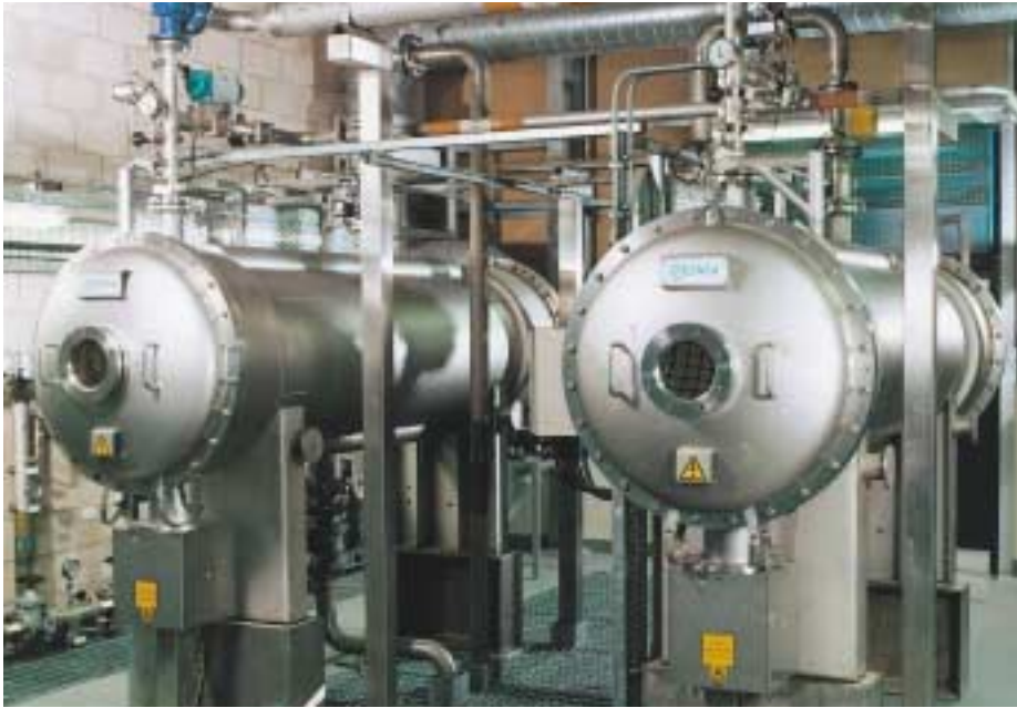
Figure 1: Headingley WTW 2 x 10.75 kg ozone/h
