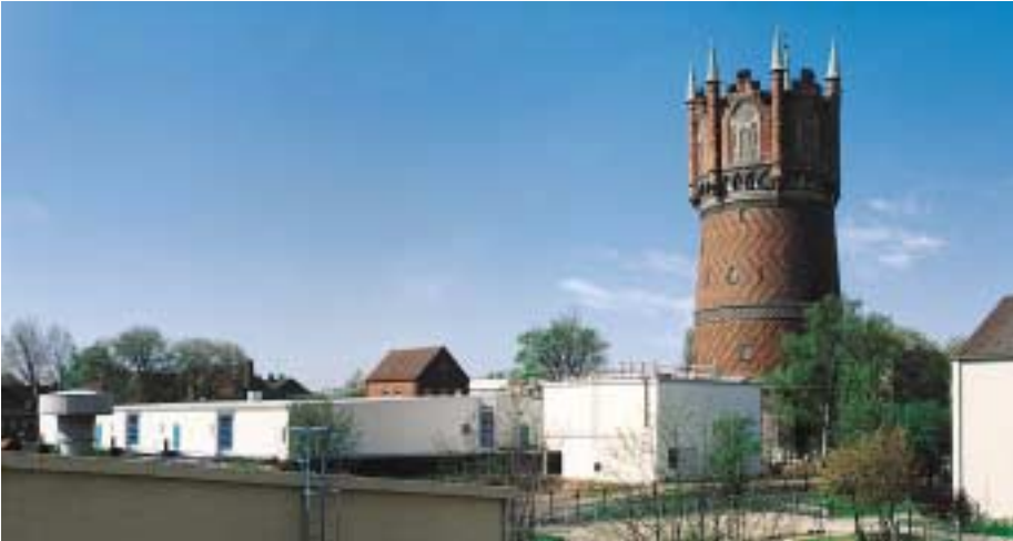
Rostock Water Works' historic water tower. In the foreground are the buildings housing the pre and mainozonation equipment.
